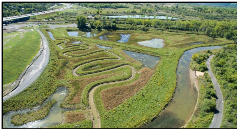
Geddes Brook Restoration Site
