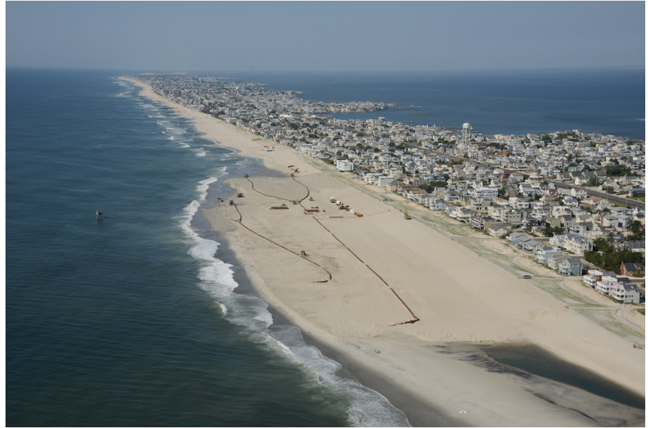
The U.S. Army Corps of Engineers Philadelphia District pumps sand onto Brant Beach, NJ in June of 2013
