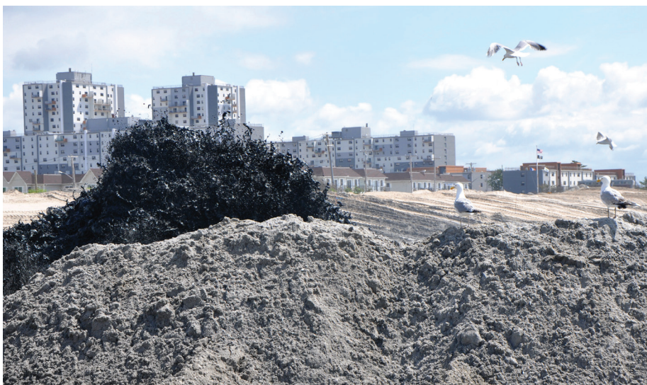
A mixture of sand and water is pumped onto Rockaway Beach, Queens, NY, June 26, 2014, from an offshore borrow site.
