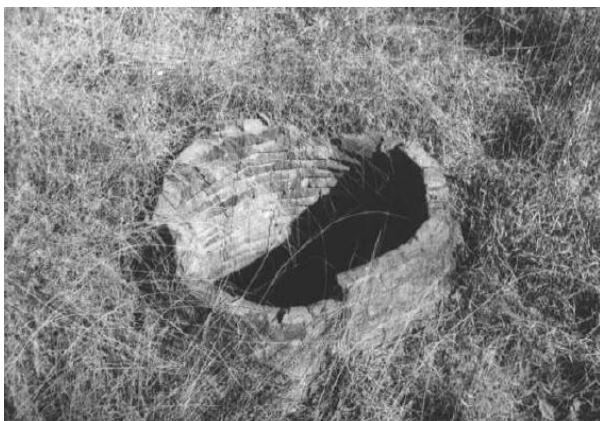
Figure 1. North Unit Cistern
