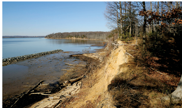
Breakwater off Mason Neck Refuge
