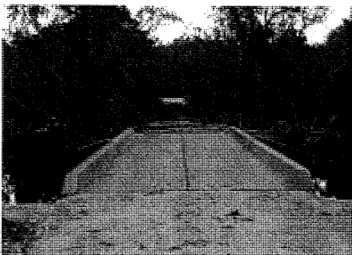
Shired Creek Bridge USFWS Ken Litzenberger
