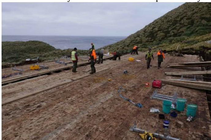
Figure 16: Helipad under construction
