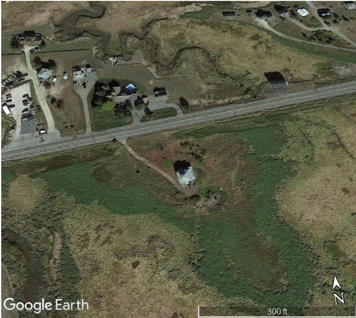
Figure 4. Aerial view of the Pink House (at center) situated along Plum Island Turnpike, Newbury, MA.
